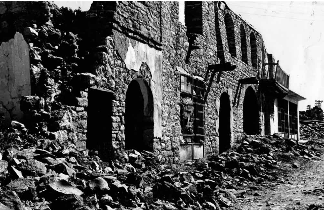
Traditional masonry housing in Lice in eastern Turkey that was damaged in the earthquake of September 1975. The old town of Lice was sited on a steep hillside (vulnerable to rock falls in any future earthquake.) The government decided to move the settlement to a new safe location, in a plain at the foot of the slope. However, this land was prime agricultural land. Further the hillside provided better protection from northerly winds than the new exposed site.
