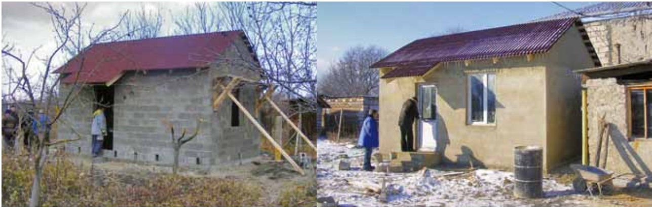
The housing strategy shifted from "one warm room" to "one warm cottage." As a result the anticipated scale of the programme was reduced Photo: Jonathan Puddifoot
